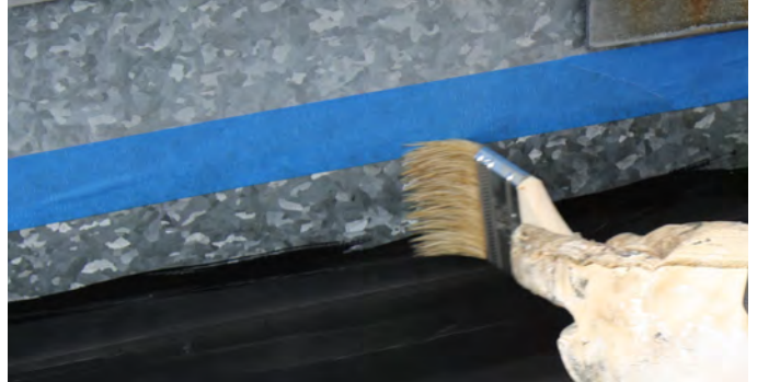
Prime all metal surfaces with M-Prime.
